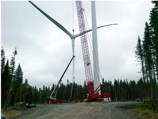
**Aug. 7, 2013-** Four [Manitowoc](#) 16000 crawler cranes are working on the Lac Alfred Wind Farm, the biggest wind farm in Canada and one of the largest in North America. Located near the village of Amqui, Quebec, the project consists of 150 wind turbines. Upon completion, the farm will have a capacity of 300 MW.
